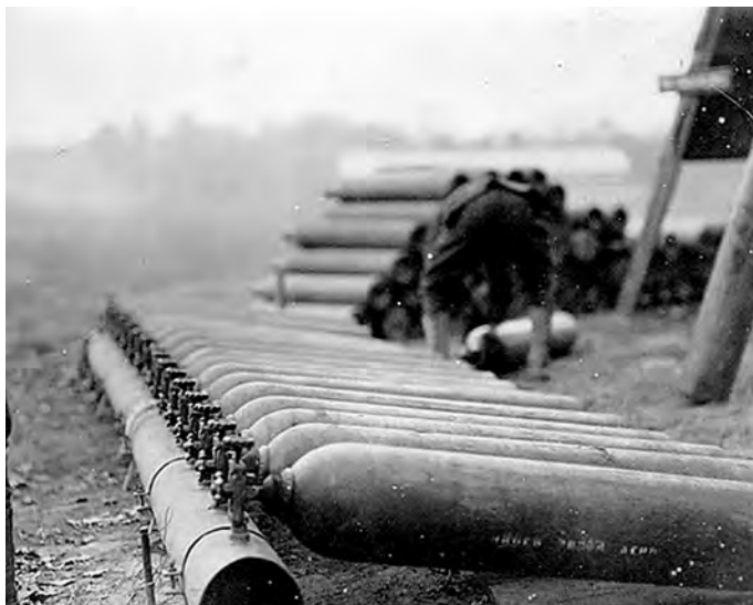
"Manifold for the hydrogen used to fill the balloons. They always leaked a little." (Photo from Camp John Wise Aerostation website.)
