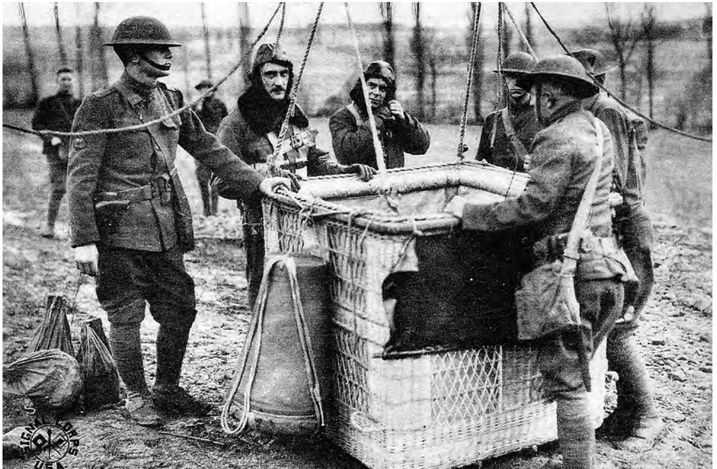
"Getting the basket ready for the observers to make their ascent." Note the parachute container just outside the basket. (Tenth Balloon Company) (Signal Corps photo 111-SC-34348, via Camp John Wise Aerostation website.)
