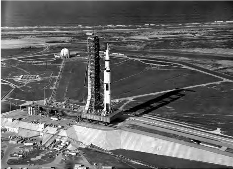
The Transporter nears the top of the five percent incline at Launch Complex 39A with the Apollo 11 Saturn V.
