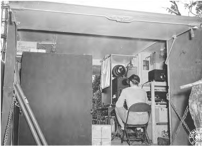
(Above) The interior of the SCR-270B operations truck with an operator at the oscilloscope. Photo taken at radar site operated by the 565th Signal AW Co., Springbrook, Queensland, Australia, Oct 24, 1942. (Signal Corps photo, National Archives.)
