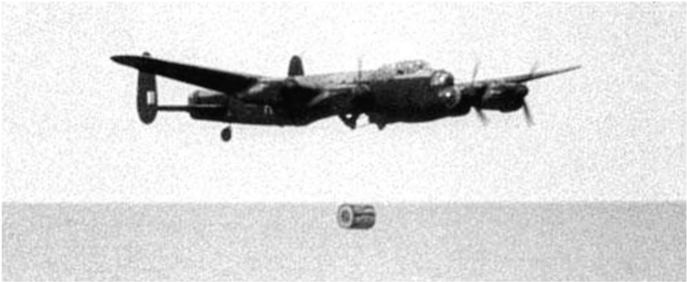
A test drop of the spinning, bouncing, dam-busting weapon for the Ruhr Valley dams.
