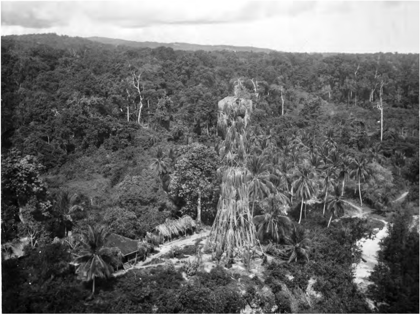
A Morotai-based US Navy PV-1 Ventura of VPB-130 imaged this IJN Type 13 radar station at Cape Mangkalihah, eastern Borneo while preparing to attack the site on January 17, 1945. This photo highlights the efforts the Japanese took to camouflage their radar sites. ( Air Force Historical Research Agency, IRIS 261620 )
