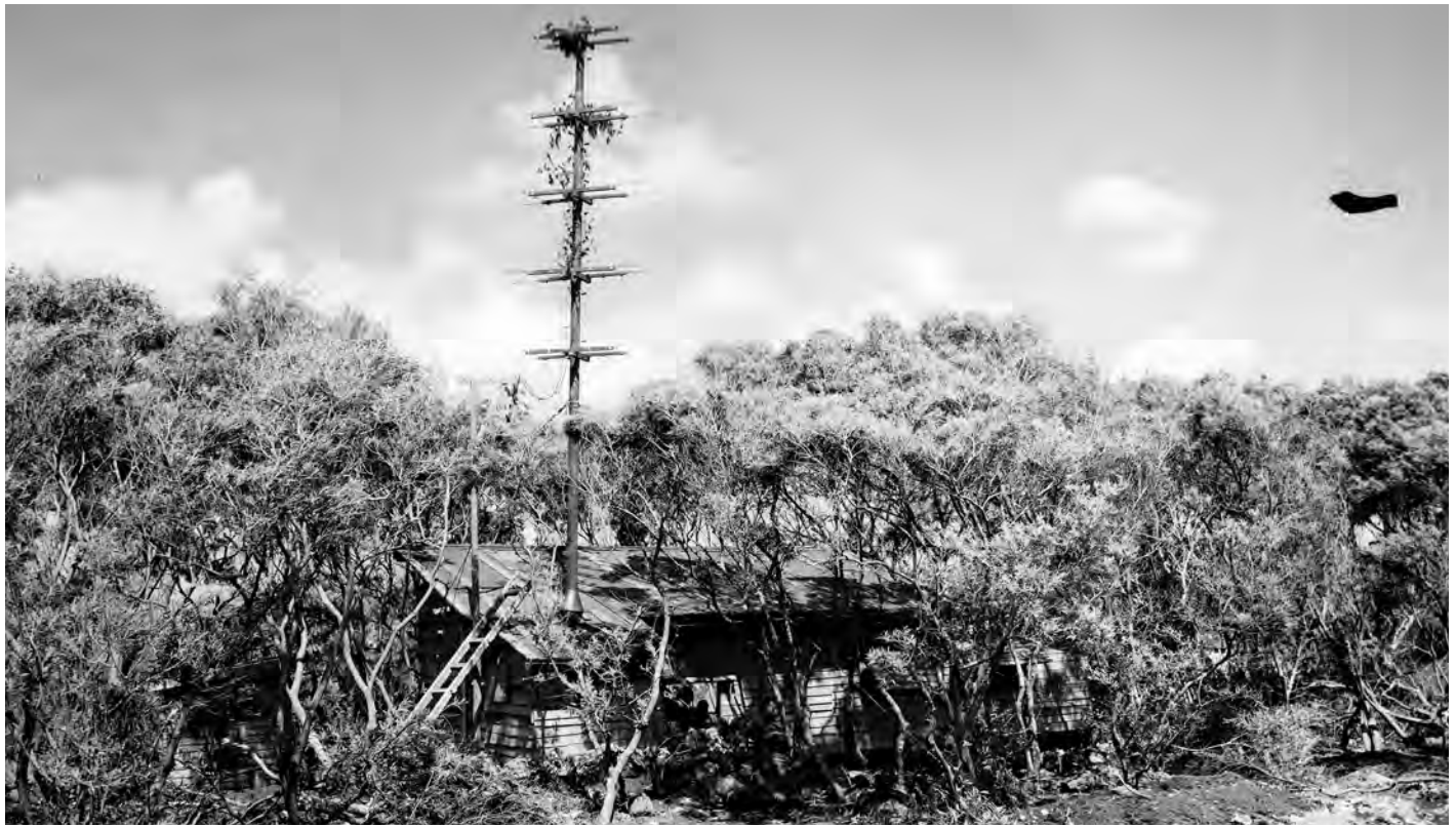
An Imperial Japanese Navy Type 13 early warning radar in a typical site hidden in the tree line. This type of deployment made precisely locating these radars difficult and led to the creation of the hunter-killer ferrets of Thirteenth Air Force. This radar was located on Saipan and was discovered during the invasion in June 1944. (US National Archives, Record Group 80-G)
