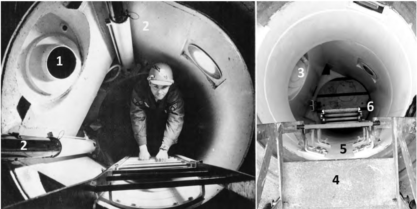
Left: Senior Airman Charles W. P. Michaels ascends PAS ladder, December 11, 1962. 1) original 22-inch autocollimator sight tube has been reduced in diameter to prevent unauthorized access. 2) the hydraulic system for opening and closing the door were originally inside the access shaft. Right: the sight tube was abandoned in place and the hydraulic system replaced with an exterior manual system during the Force Modernization program. 3, 4, 5) are the portable, fixed and extension ladder sections respectively. ( Library of Congress )
