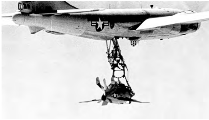
The XF-85 Goblin hangs under a B-36 in its trapeze.
