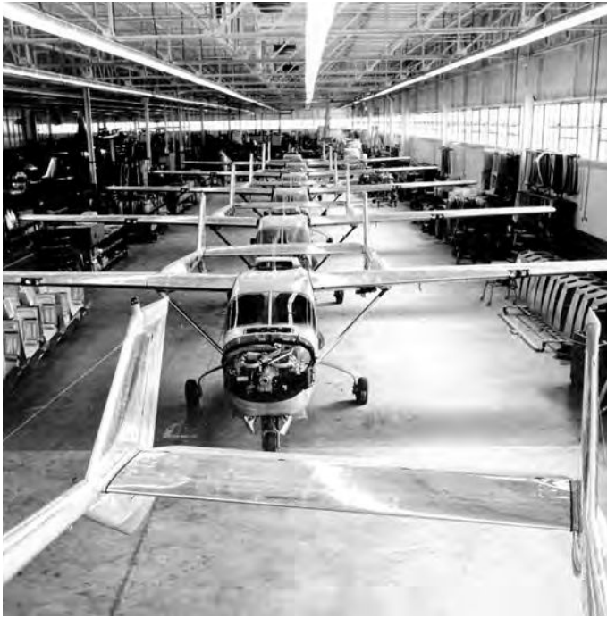
Cessna O-2 Assembly Line Wichita, Kansas, date unknown. (Photo courtesy of the Kansas Historical Society.)
